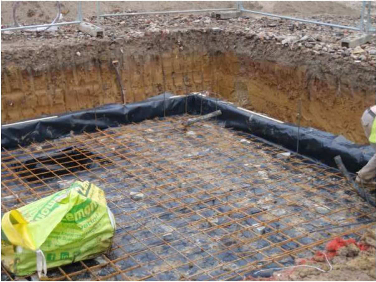
Plate 6. Main inverter building under construction (looking north).
