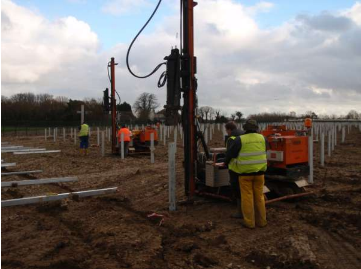
Plate 5. Piling in progress
