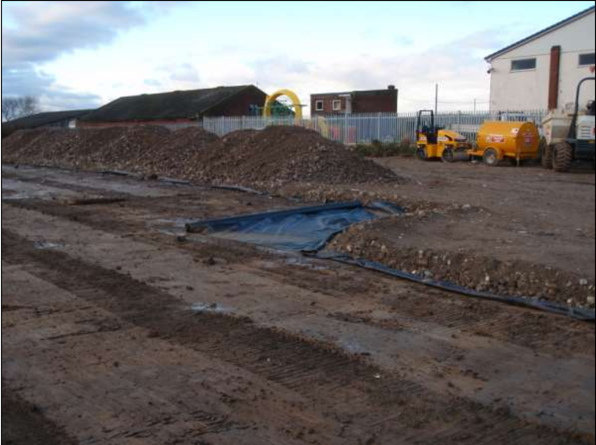
Plate 2. Construction compound being built (looking east)
