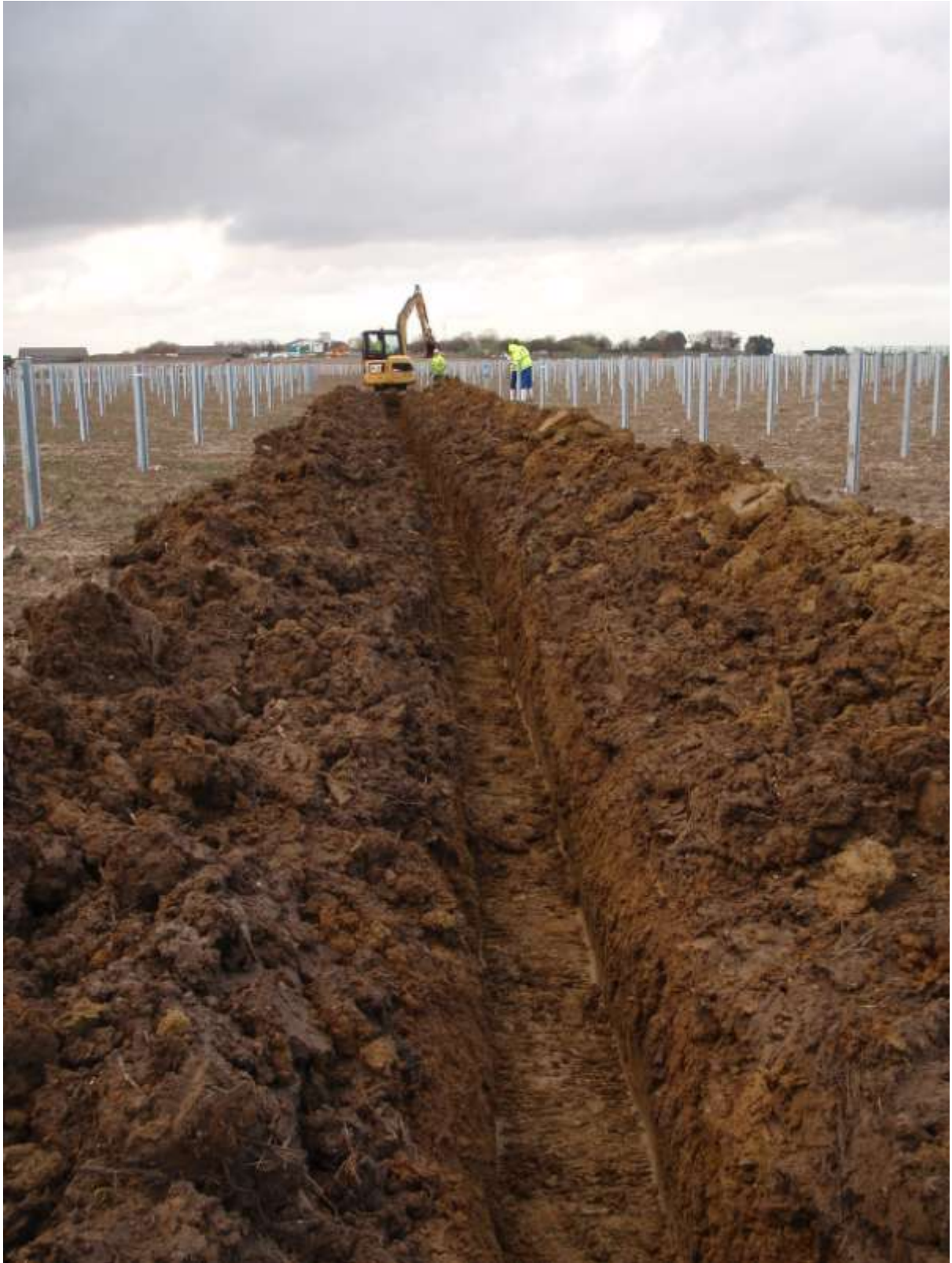
Plate 4. Main cable runs excavated with ditching bucket (looking south)
